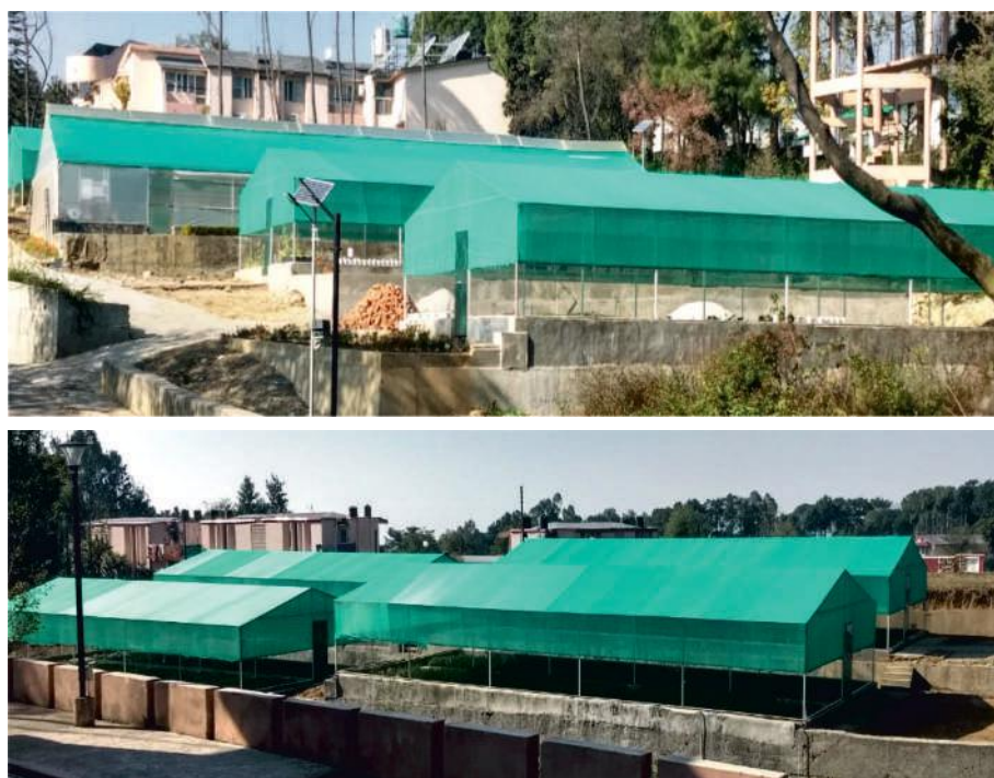
Net and Poly Houses facilities
