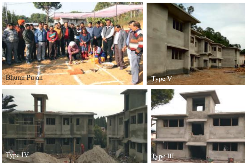
Bhumi Pujan and construction of Type V, IV and III quarters
