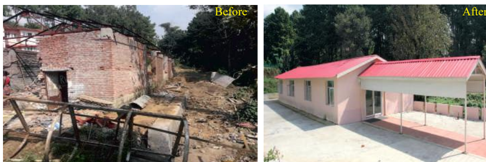
Community Hall before and after construction
