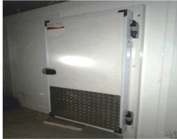
Cold Storage facility
