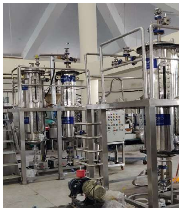
Fig. 4 Installation & commissioning of DBT-BIRAC funded Separation columns.
