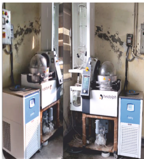
Fig. 3 Installation and commissioning of DBT-BIRAC funded Solvent recovery system.
