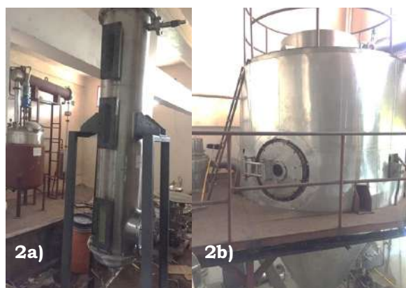
Fig. 2 Design and Installation of a) Stainless steel adsorption column & b) Spray dryer at Company site.
