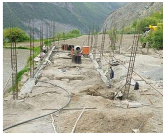
CFC Construction site of Shansha cut-flower cluster
