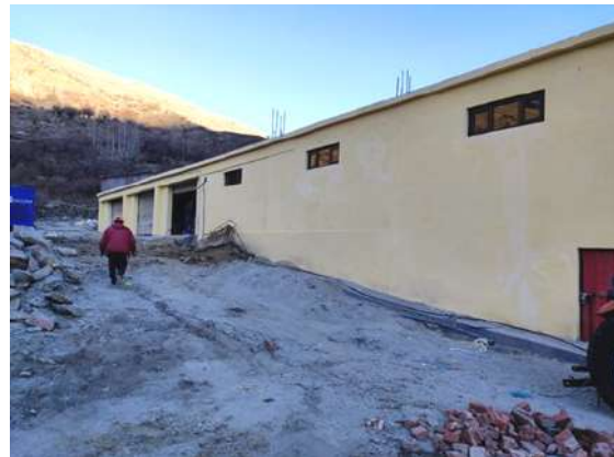
Common Facility Centre (Gondhla Cut-flower cluster)
