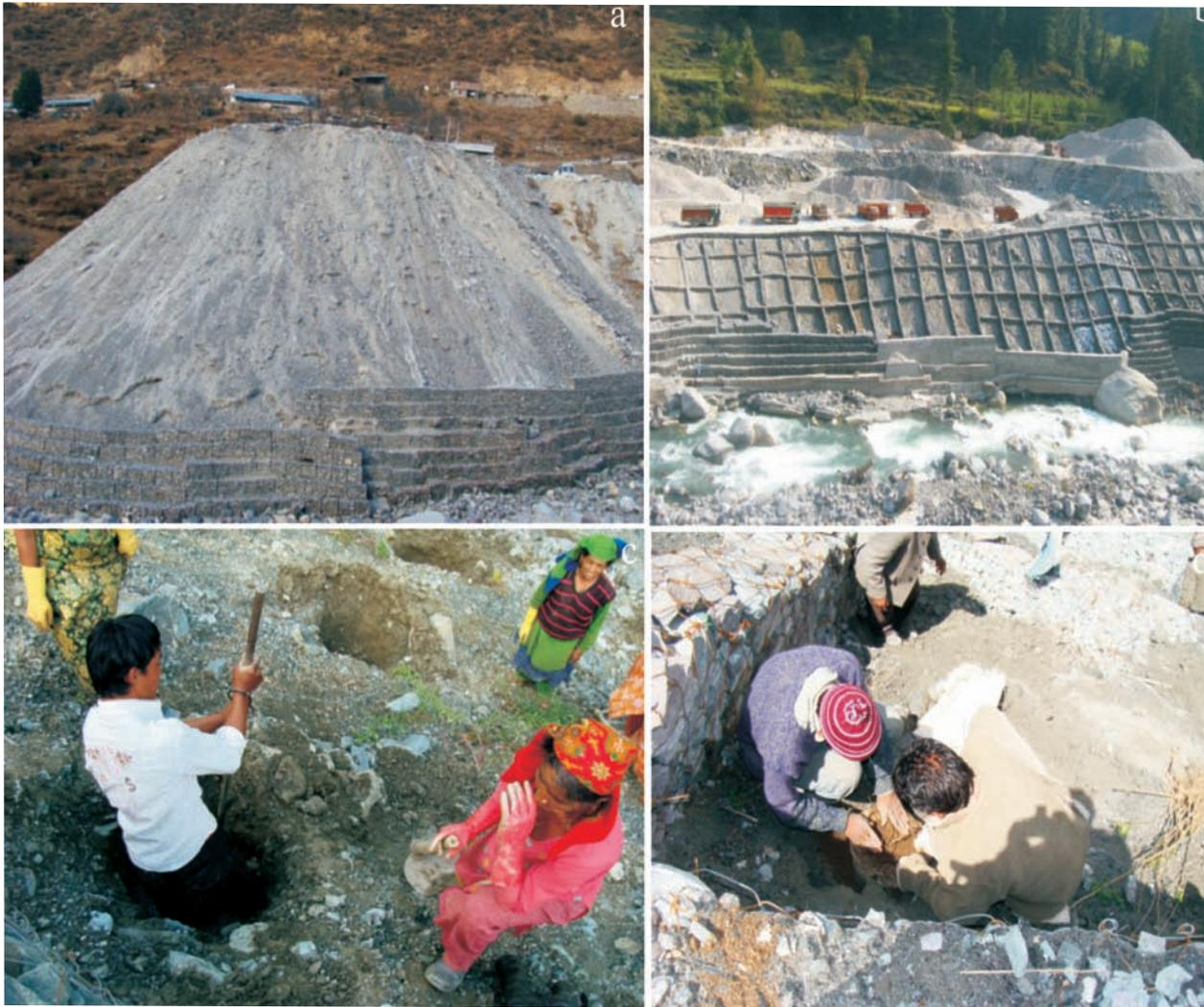
Fig. 7 Revegetation a) closed dumping site, b) muck-dumping site, c) digging of pits, and d) planting of saplings
