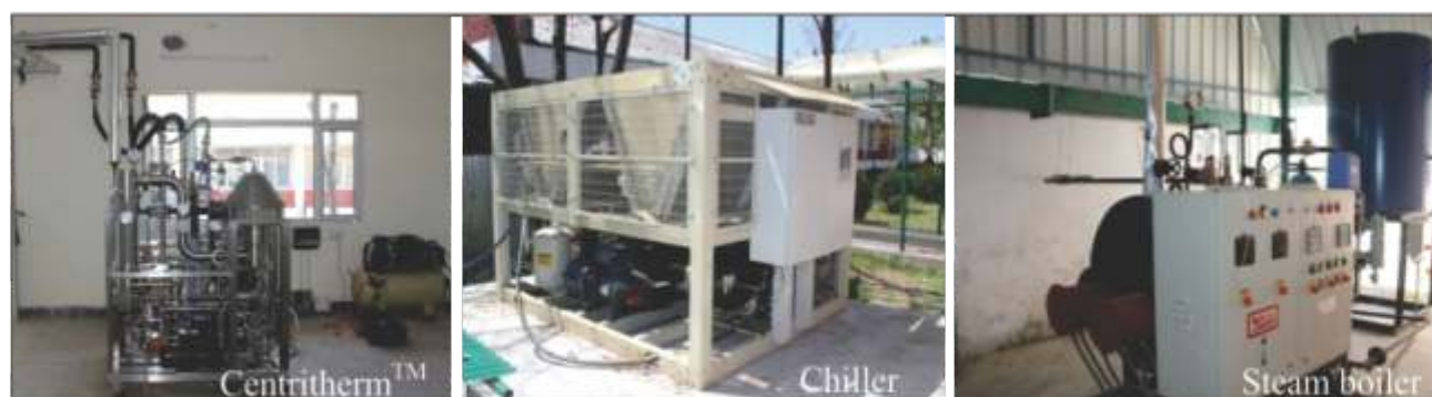
The pilot scale thin film, spinning cone evaporator installed at CSIR-IHBT
