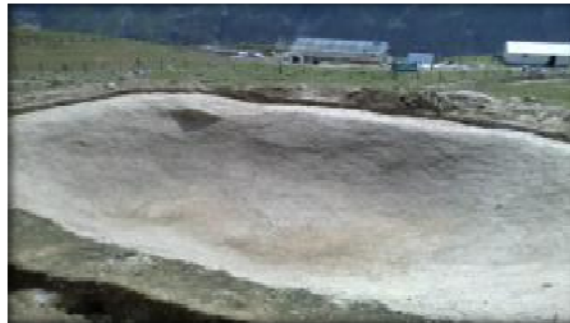
Demonstration of snow Water harvesting
